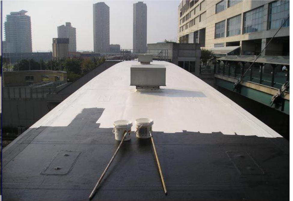
Ceramic InsulCoat Roof can be applied via brush, roller or sprayer
