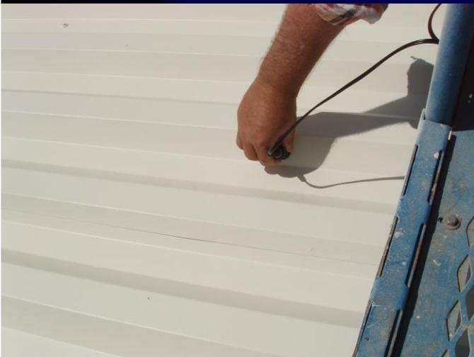
A series of Ultra-Sonic readings are taken to measure dry film thickness
