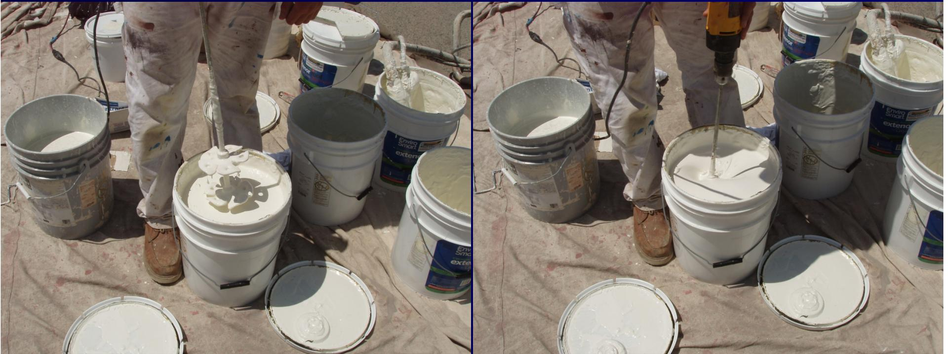
Drill Paint Mixer used to Stir Product On-Site
